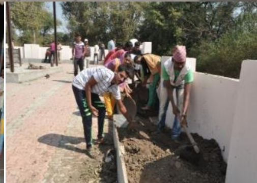
Nala cleaning and village survey in Nandoshi Village by NSS Volunteer
